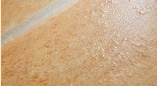
TI (tiles) – tile appearance with original joint pattern
